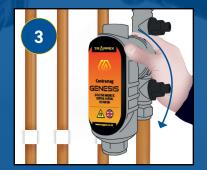
Replace magnet and turn it 180 degrees. Re-tighten collar.
