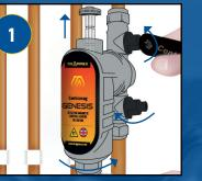
Isolate both valves, remove magnet, open drain plug and drain.
